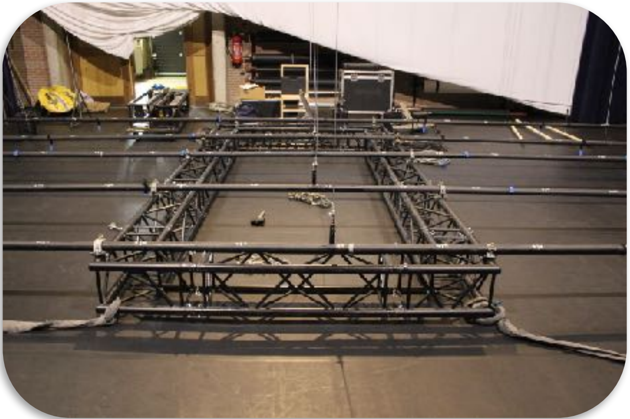
OPTION 1: The truss frame, directly attached to the fly system of the theatre.
